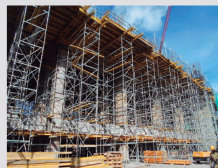
GRAND HYATT (Bogotá) Sistemas Empleados: ST-100, Multiflex, PEP Ergo y Peri Up.
