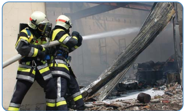
In this warehouse fire in France, the firefighters were able to shelter behind the concrete wall in order to approach the fire closely enough to extinguish the flames. Courtesy of DMB/Fire Press.
