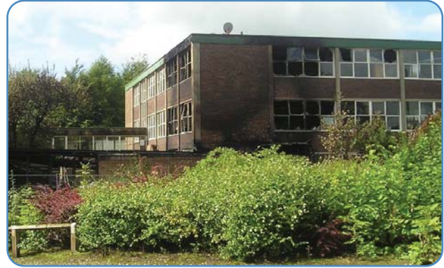
The impact of a major fire at Tytherington County High School, Cheshire was limited due to the fire resistance of the concrete structure. Rather than taking a year to be demolished and replaced, as was the case with an adjacent lightweight structure, the concrete classrooms were repaired ready for the following term.
