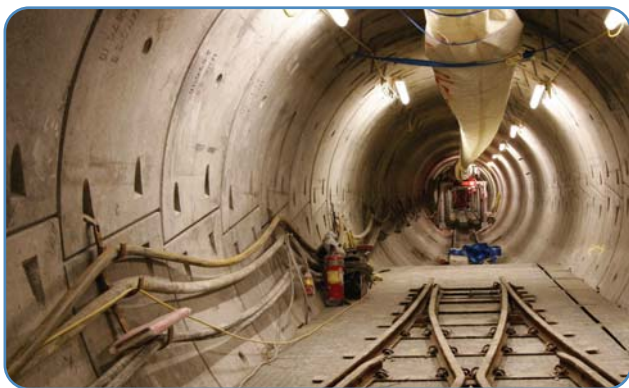
Tunnel fires can reach extremely high temperatures, therefore concrete is a good choice for tunnel linings. Courtesy of Tarmac.
