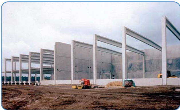
Precast walls form fire resistant compartmentation for this storage facility. Courtesy of BDV.
